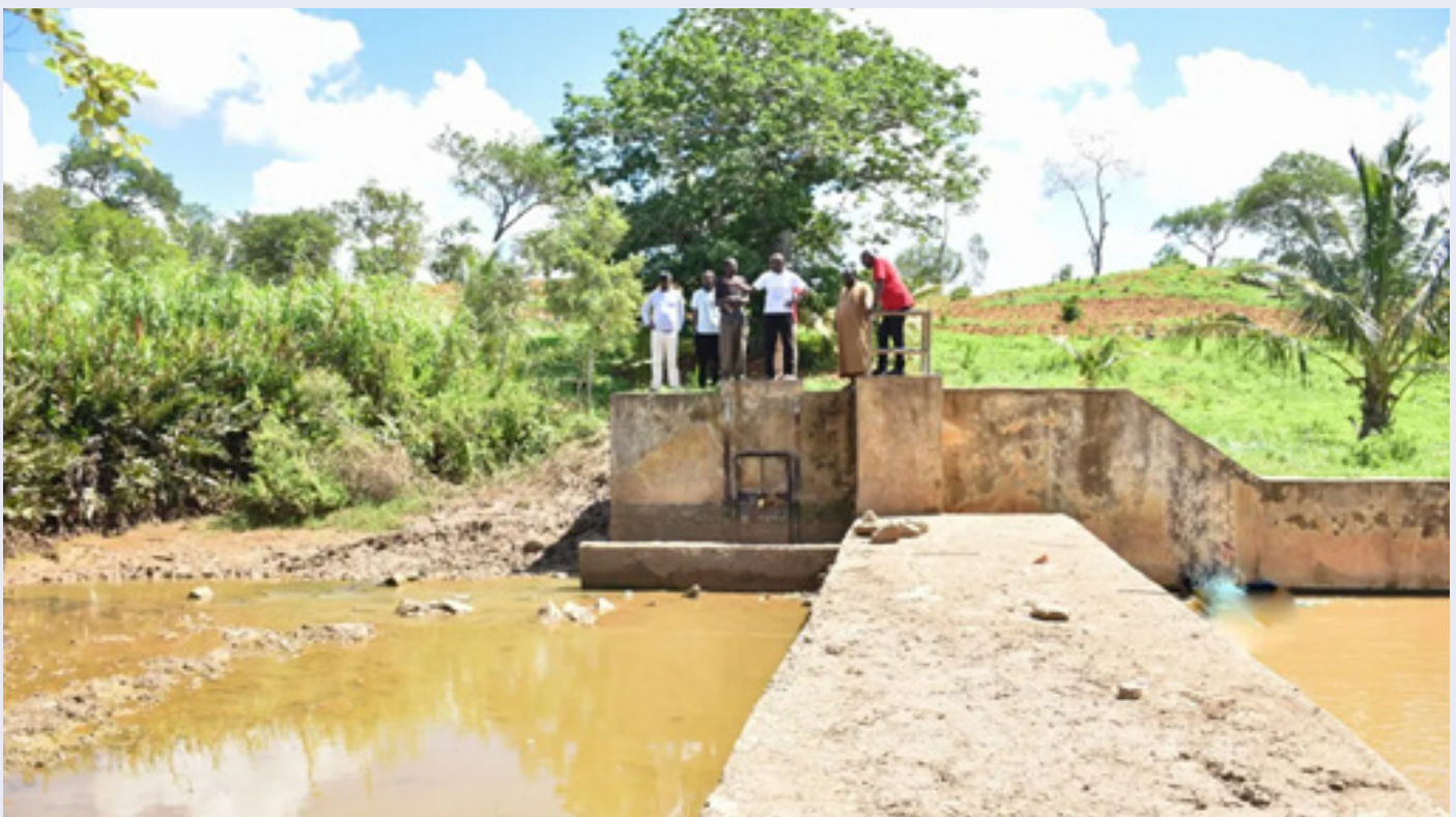
Mdachi Irrigation project
